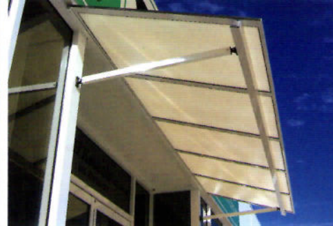
Above: 50 x 50 beam for larger arm spans
